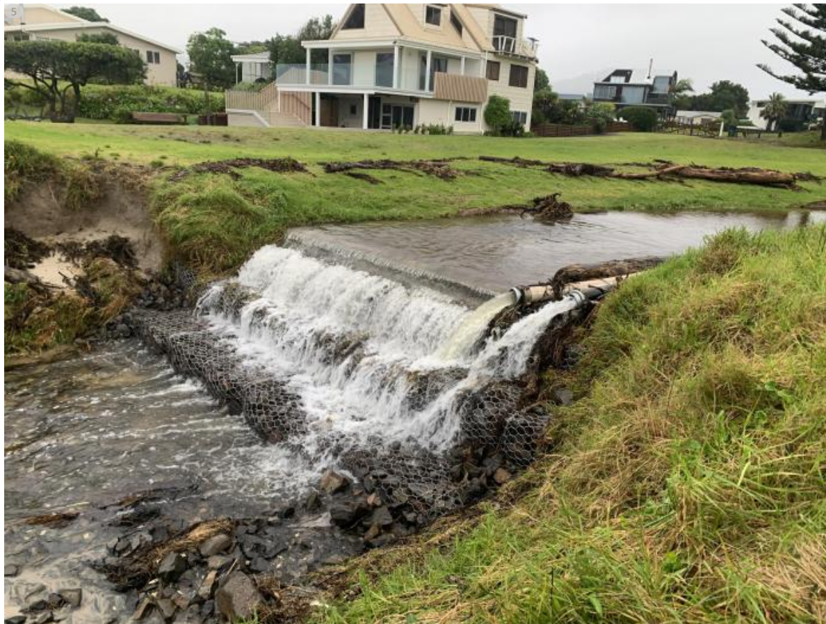
105 Weir at 13 March with pumps running.jpeg
