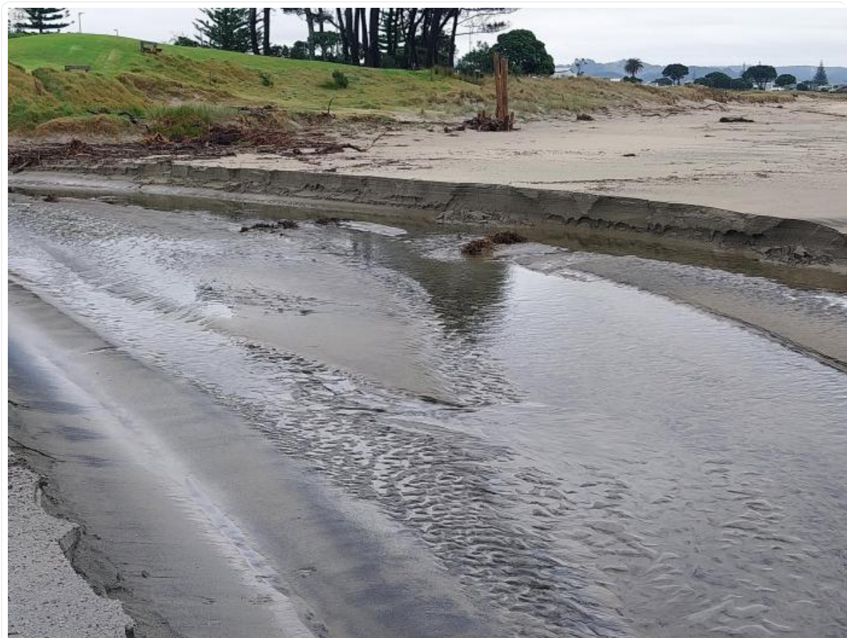
141 erosion of beach into channel 20230618_090914.jpg
