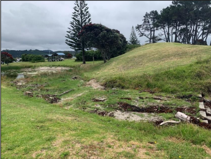
Figure 4: Overflow channel from pond to weir
