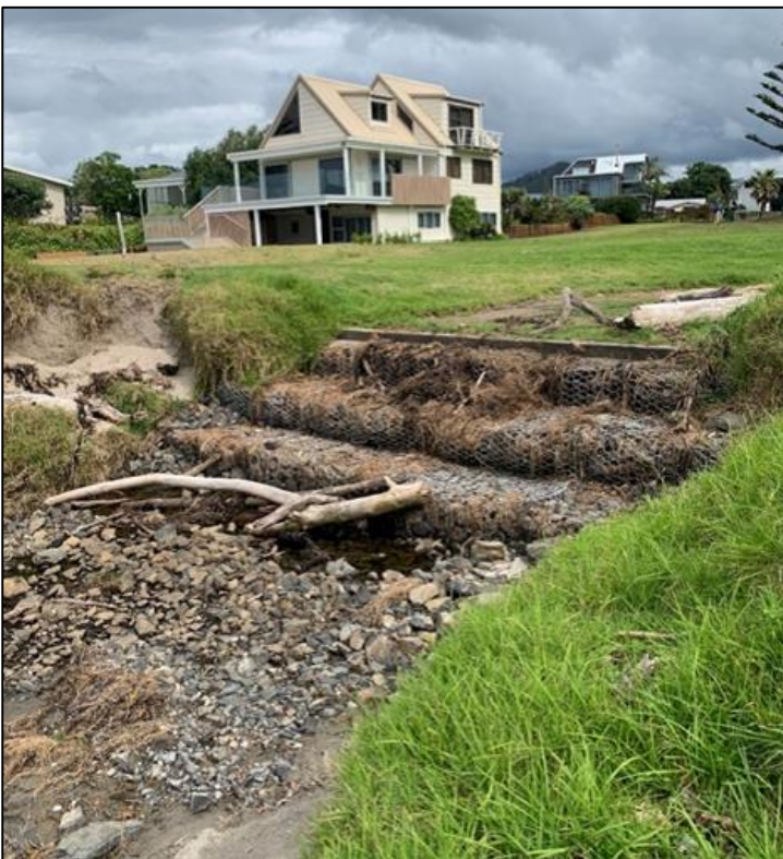
Figure 5: Existing weir and gabions
