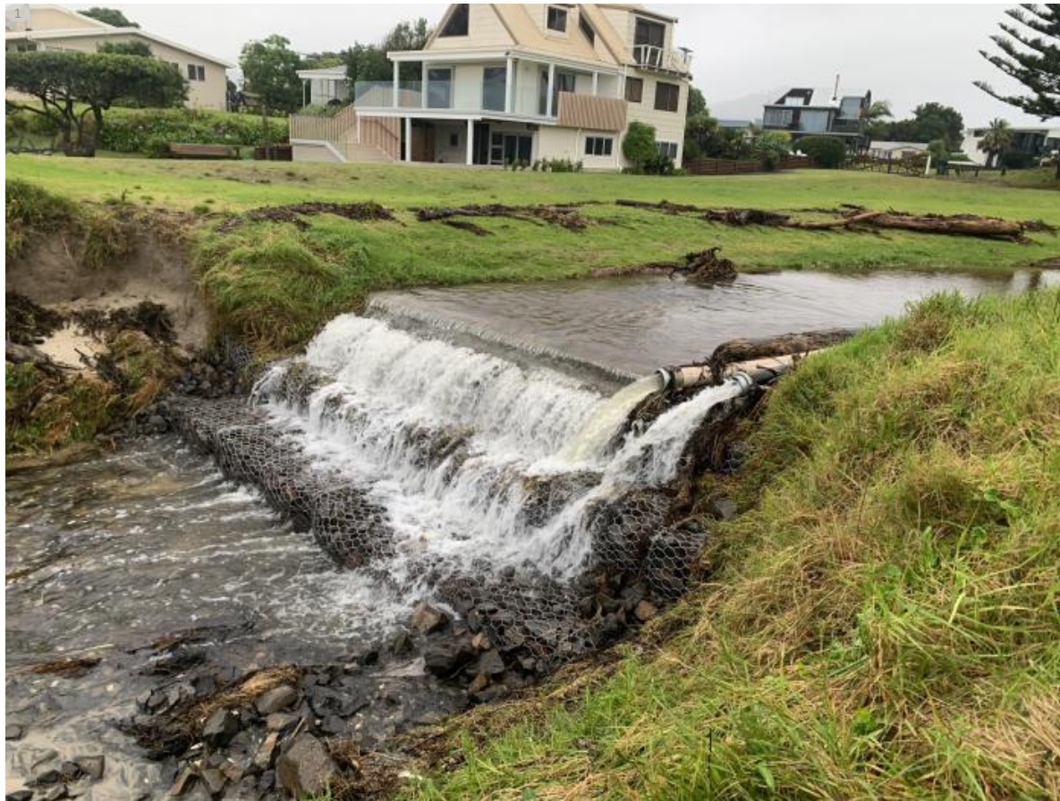
105 Weir at 13 March with pumps running.jpeg
