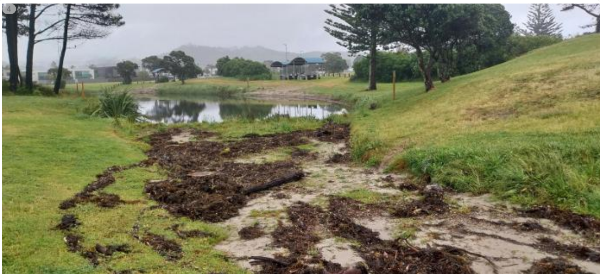
130 King Tides breached weir 1 November 2023.jpg
