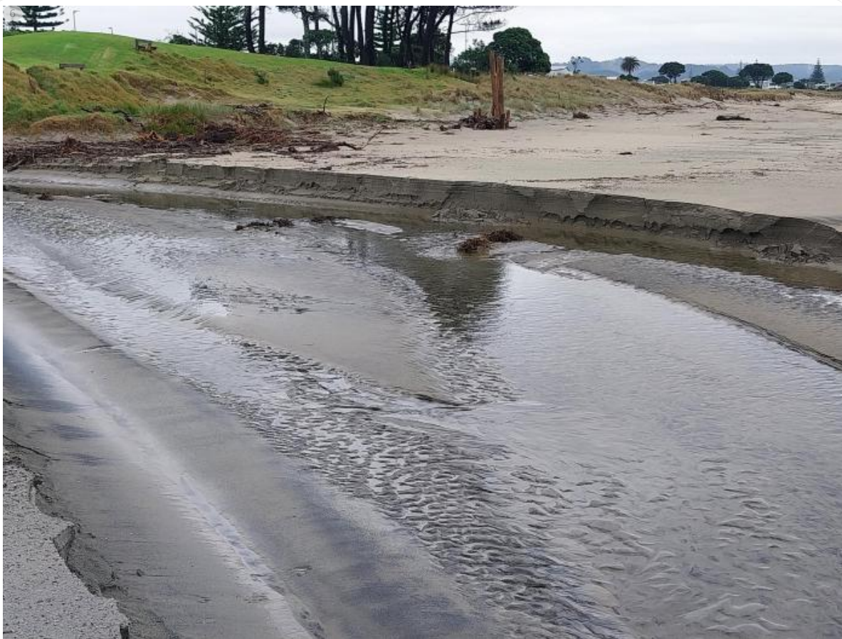
141 erosion of beach into channel 20230618_090914.jpg
