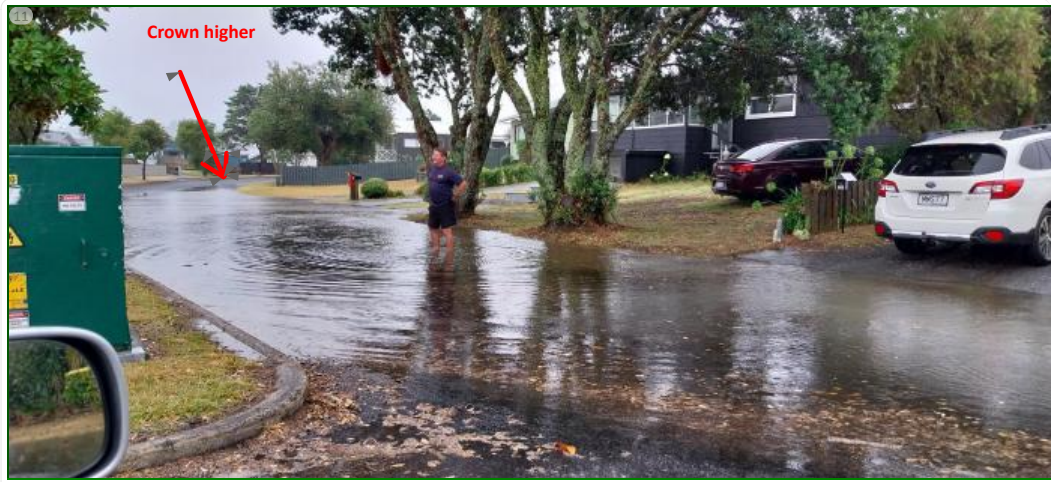
20240222 Chartwell sumps clear but not draining.jpg
