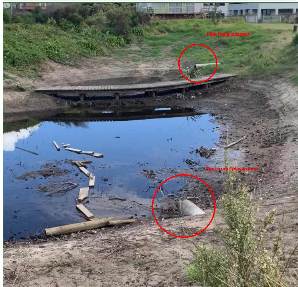
174 mp4 showing both pipes.jpg
