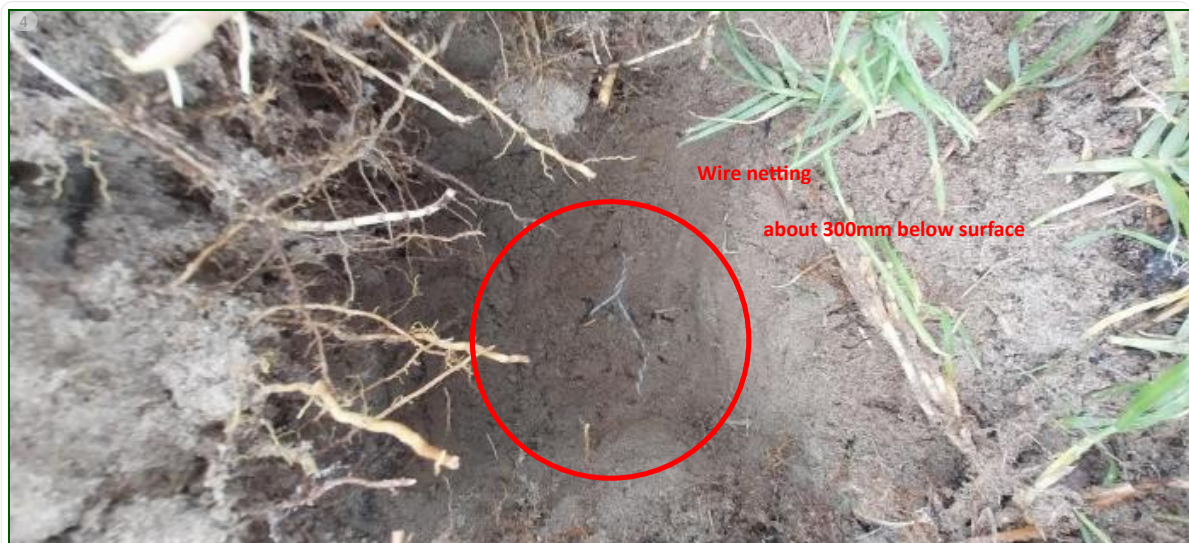
030 Wire netting about 300mm below surface 20240404_161314.jpg
