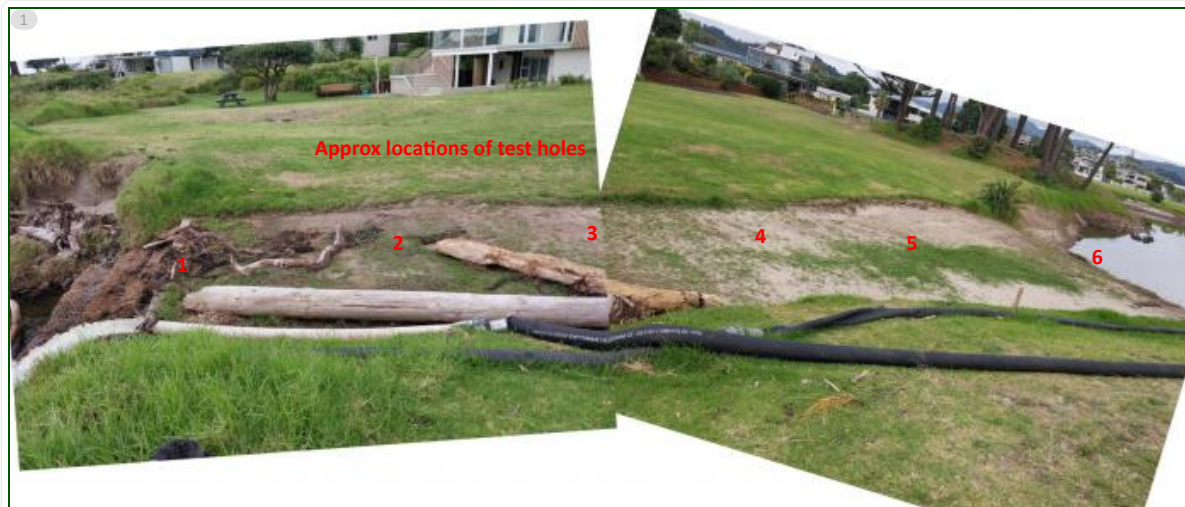
001 weir spillway 20240404_172911_SC_.jpg
