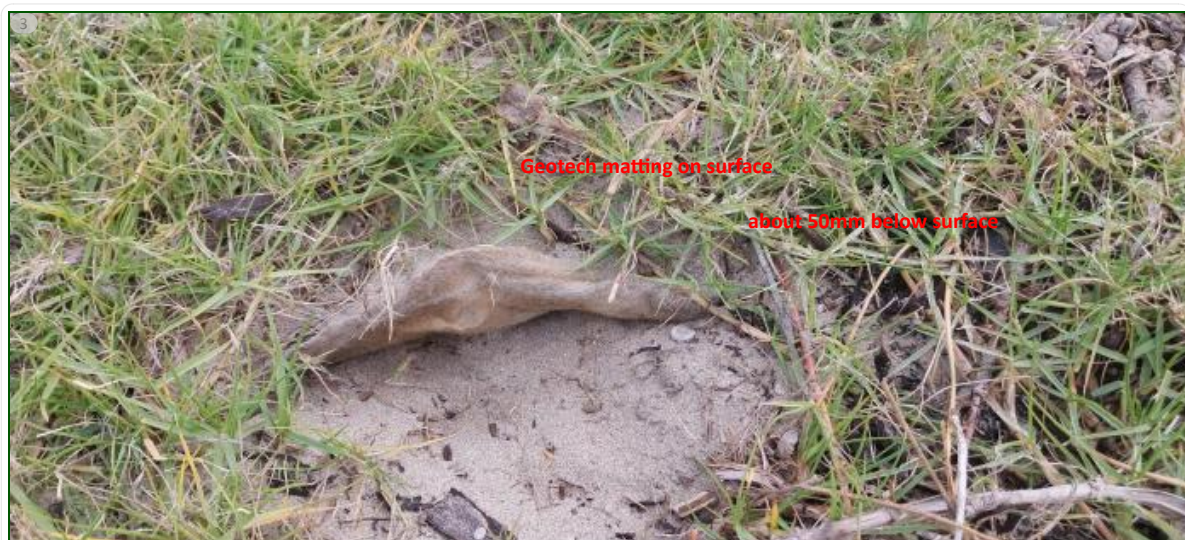
020 Geotech matting 20240404_161140.jpg
