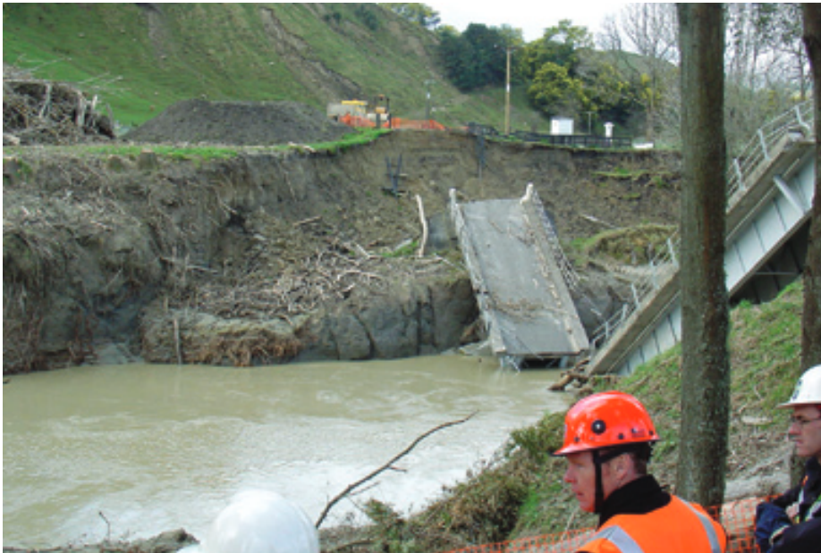
Mangamahu Bridge (Lower North Island floods, 2006). Photo courtesy of Ministry of Civil Defence and Emergency Management
