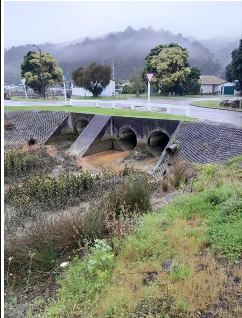
June 2022 Burke Street Outfall
