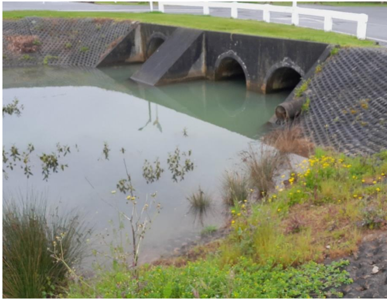
Ref 03 February 2022, Burke Street Outfall
