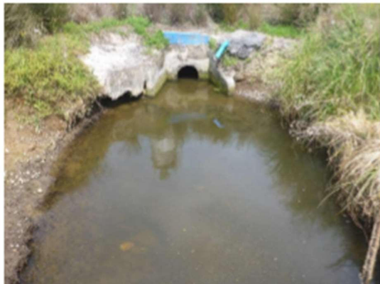
Photo 13. Site 13: Lindsay Rd, Whangamatā.
