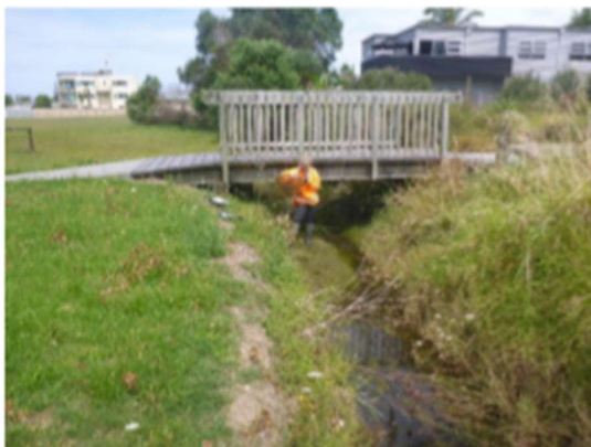
Photo 10. Site 10: Casement Rd, Whangamatā.
