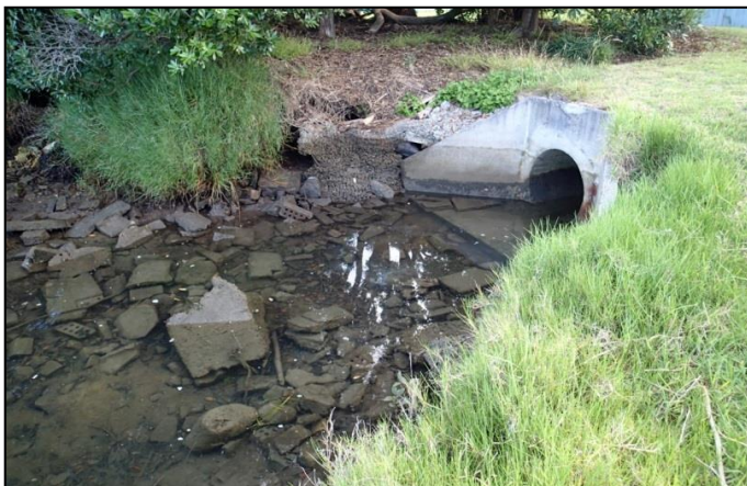
Photo 7. Site 7: Marquet Place, Tairua Harbour.
