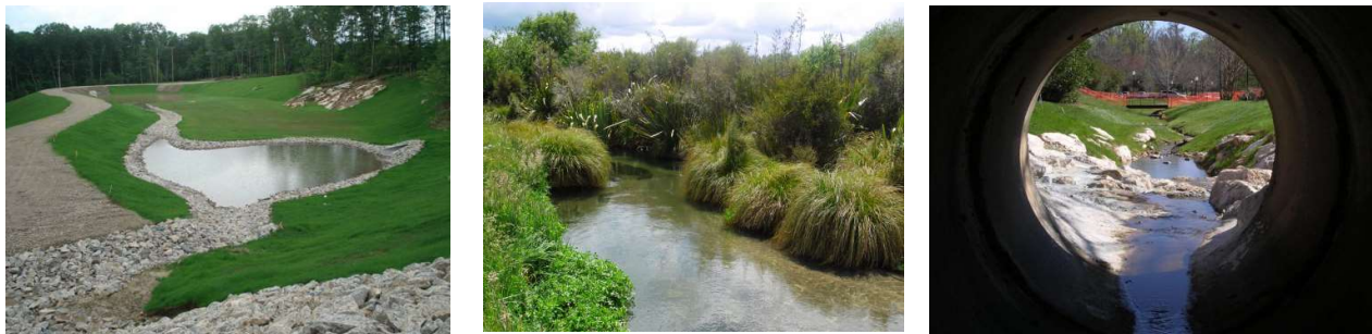
Figure 9 – Examples of stormwater infrastructure around New Zealand. The first photo shows a detention pond with energy dissipation. The second photo represents riparian planting along a riverbed. The third photo shows a perspective from inside a stormwater outfall.
