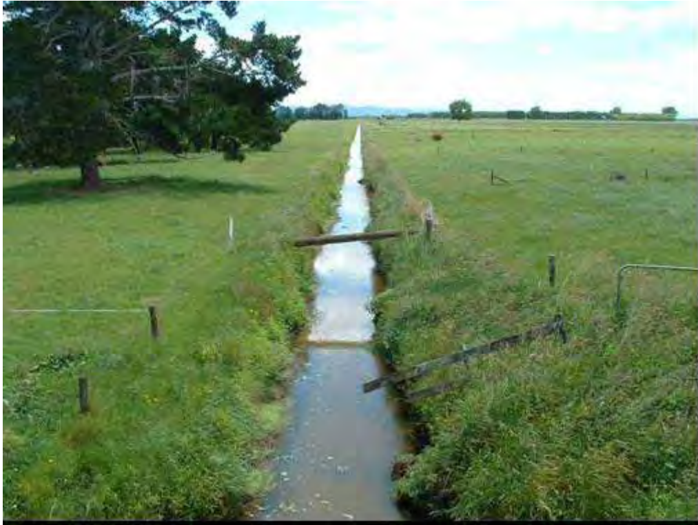
Photo 10 Conventional open ditch peat drain
