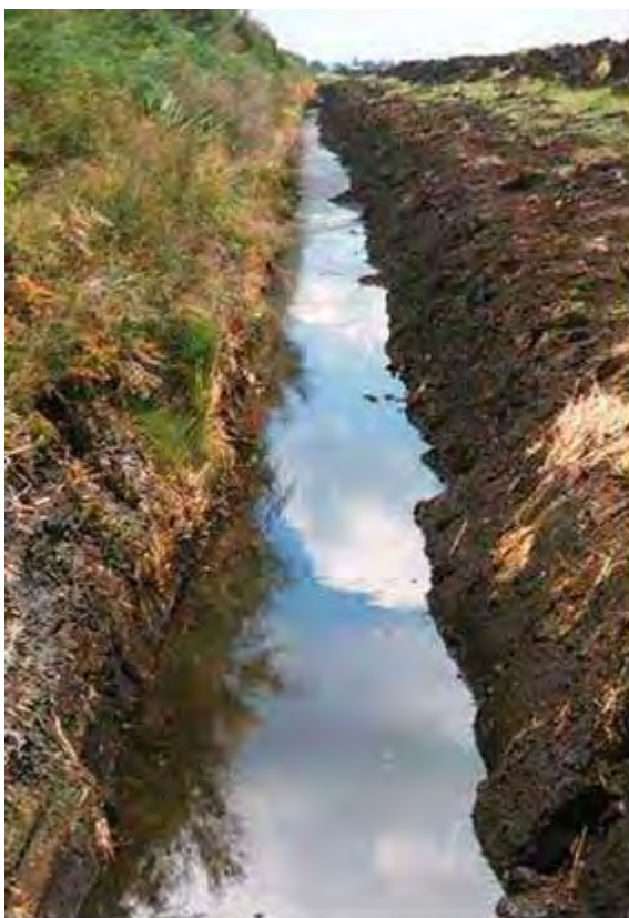
Photo 12 Excessively dug drain
