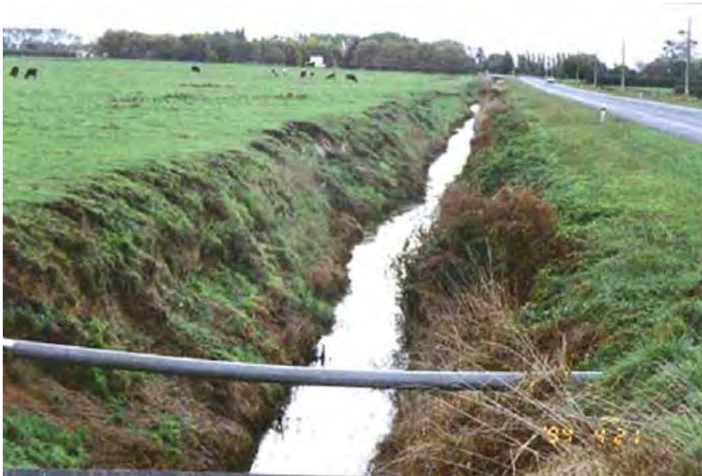
Photo 5 Drain bank erosion caused by stock
