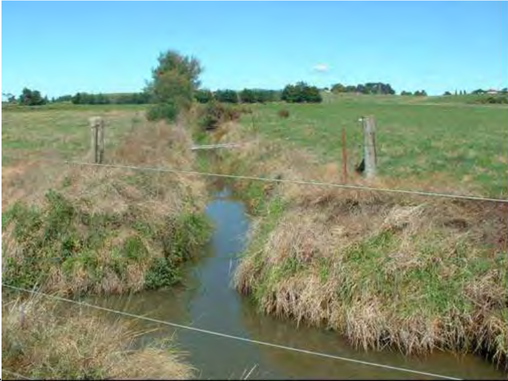
Photo 7 Fencing constructed close to the drain to allow space for an excavator to reach over the top and undertake maintenance if required.
