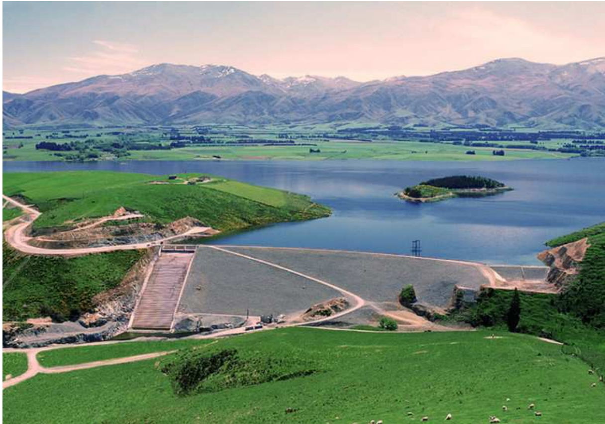
Figure 6-6: Opuha Dam showing the dam wall and spillway with the lake behind. The deepest part of the lake lies between the island and the dam wall. The monitoring tower is visible in the lake near the middle of the dam wall. [Internet media photo].
