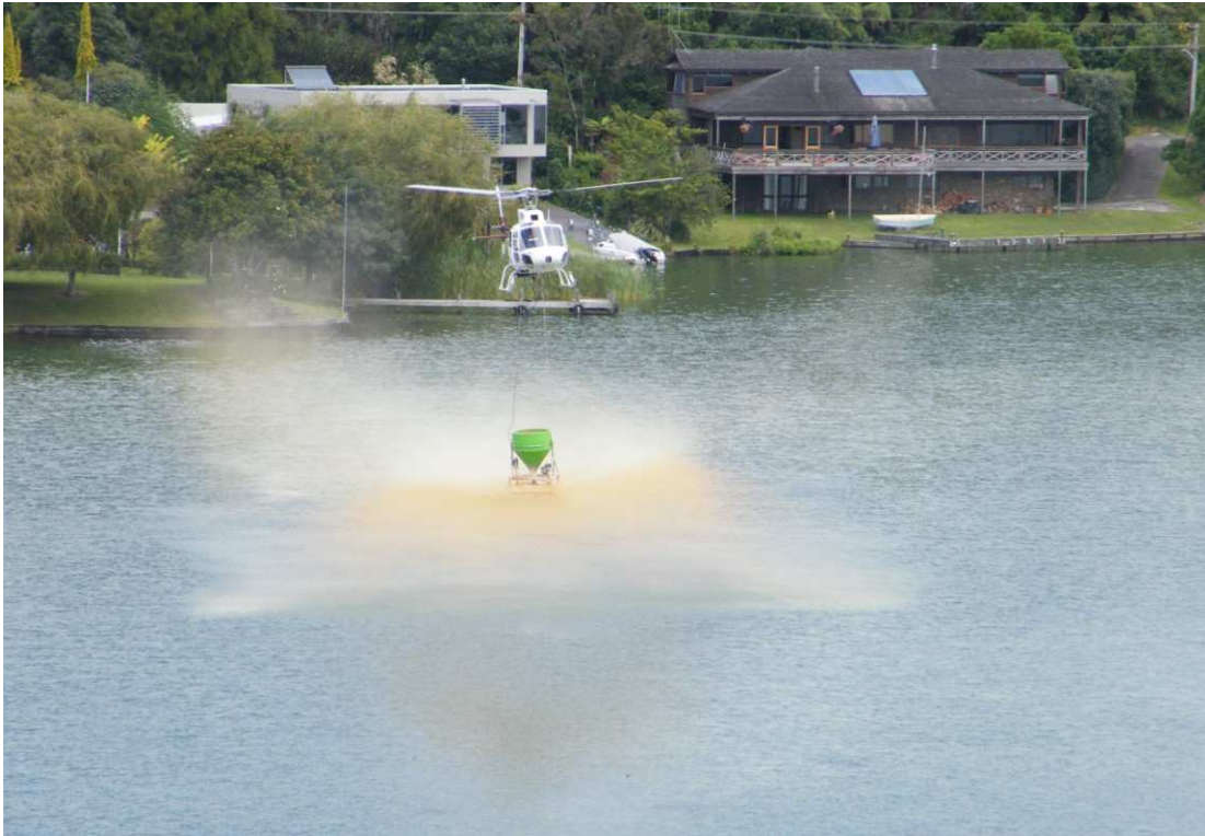
Figure 5-13: Application of Aqual P TM as a slurry from a helicopter on Okawa Bay, Lake Rotoiti. The helicopter position was controlled using GPS navigation. [Photo: Graham Timpany, NIWA, Rotorua].
